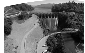
Ruskin Dam – Right Abutment Seepage Control Upgrade Golder Construction Inc.
