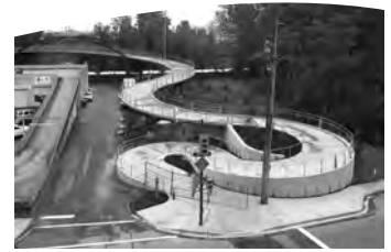
Harbourside West Pedestrian Overpass Hatch Mott MacDonald
