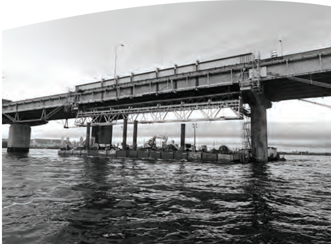
Design and Construction Engineering of the Champlain Bridge Superbeam and Modular Truss Buckland & Taylor | COWI
